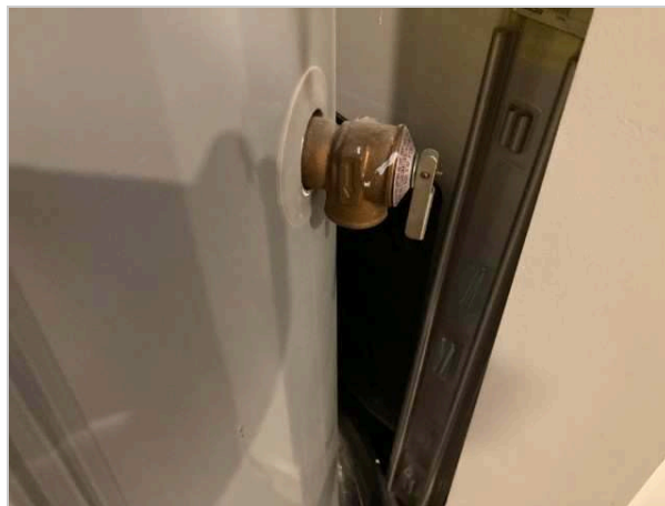
Missing discharge pipe
