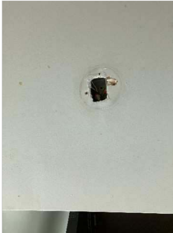
Exposed wires
